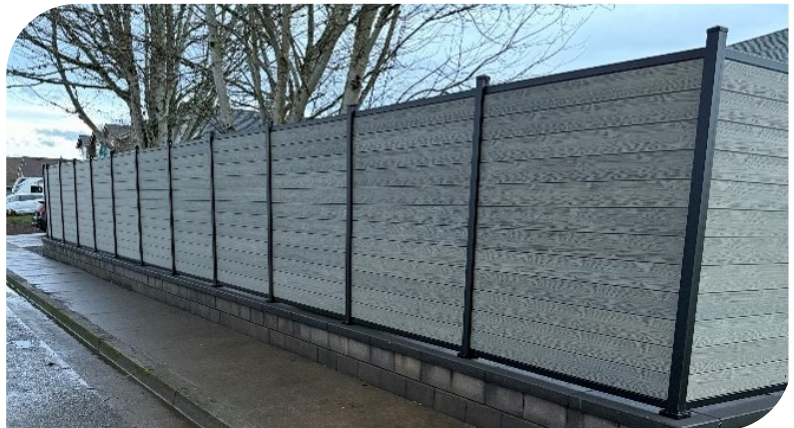
Figure 7. Minor renovation in Polk County.
